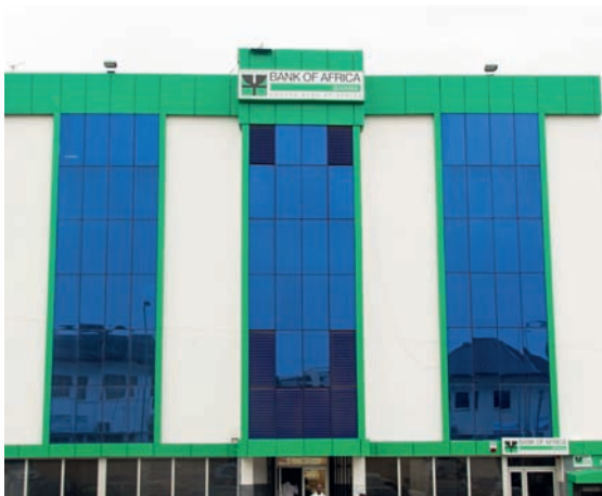
BOA-GHANA: Head Office Building, in Accra.
