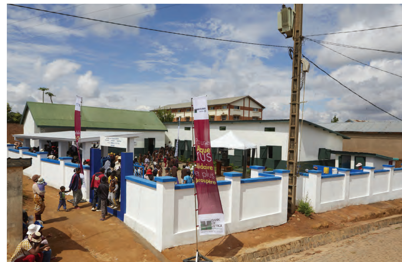
Renovation of a primary school
