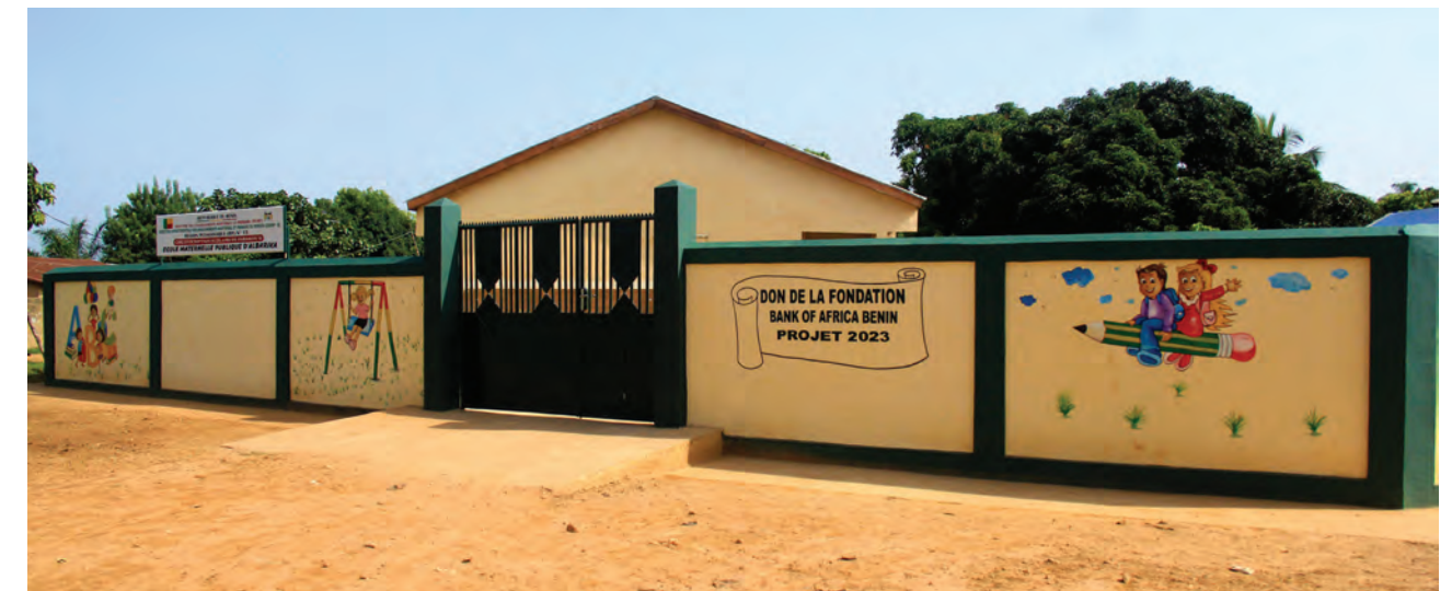
Renovation of Albarika nursery school in Parakou
