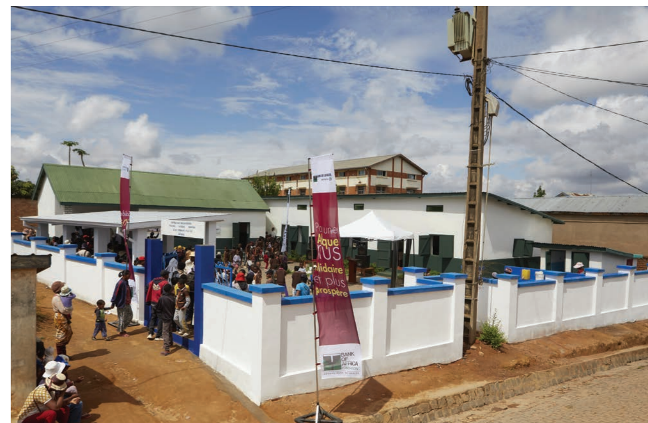
Renovation of a primary school
